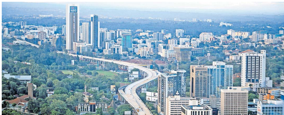
The Nairobi Expressway. While the growth rates the country has been posting have been respectable, that growth has been increasingly debt-financed and in unproductive sectors.
